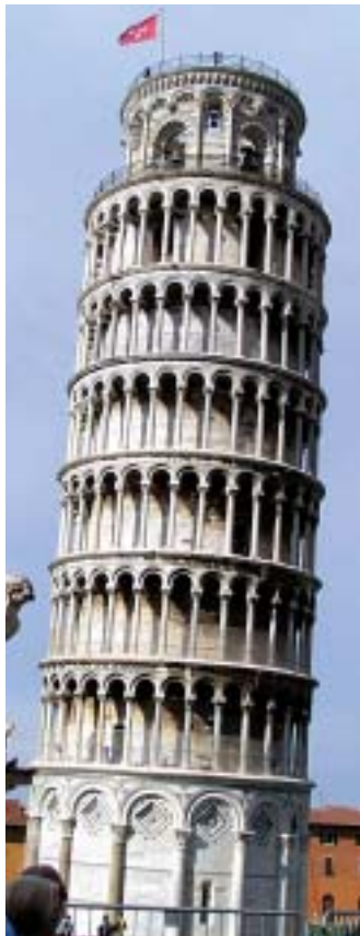
LEANING TOWER OF PISA
