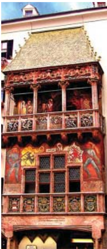
GOLDEN ROOF - INNSBRUCK
